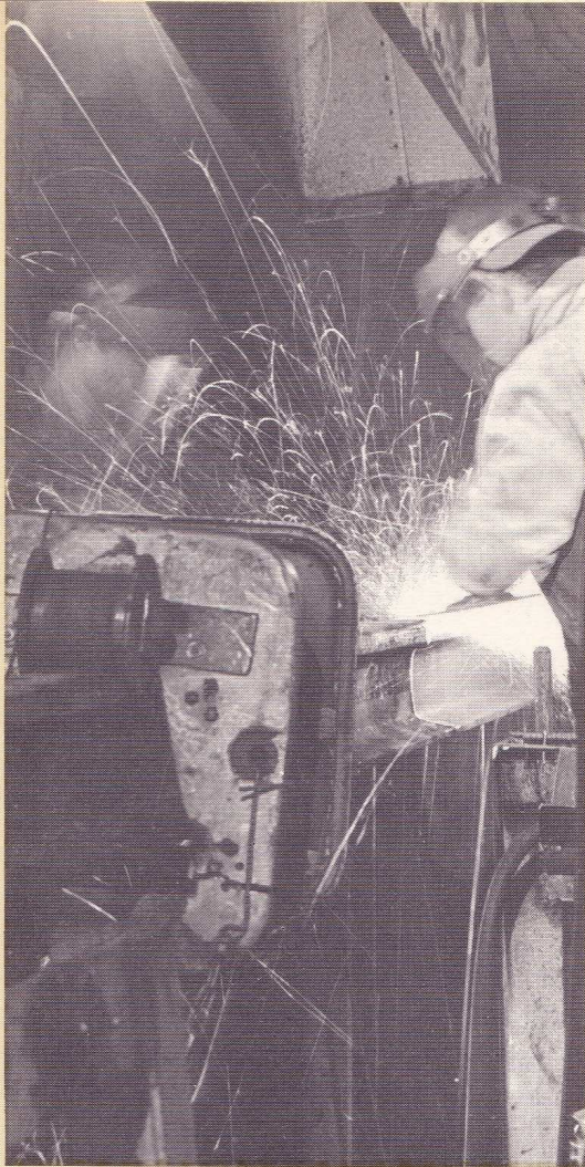
New rail sections being welded together in quarter-mile lengths.
