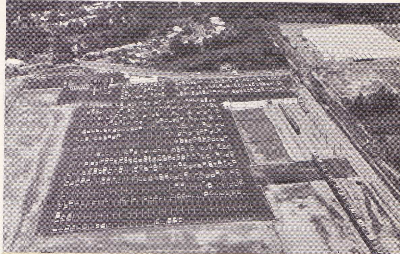
Friscos newly-constructed automobile and truck facility at Memphis, Tenn. Spread out over 47 acres and paralleling the railroad's main line, this site has storage accommodations for 1200 vehicles, the largest such facility in the South.
