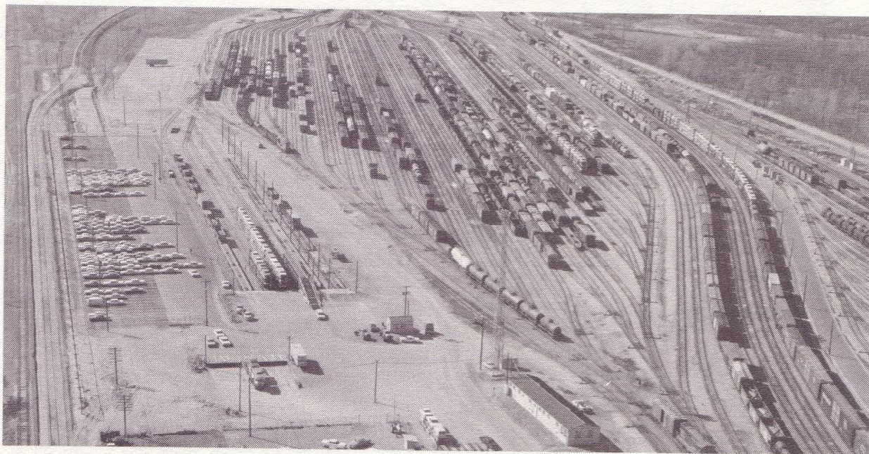
Aerial view of Frisco's push-button yard at Tulsa, Oklahoma.
