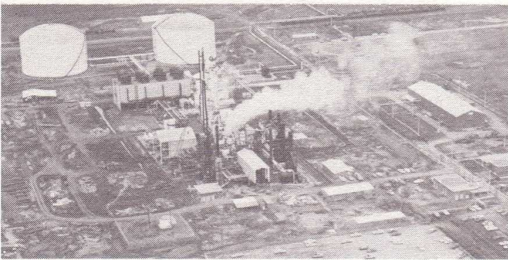
Continental Oil Company's new plant now under construction at Armorel, Arkansas.
