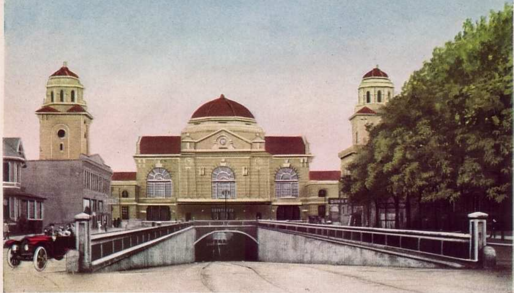
5363. Terminal, Birmingham, Ala. SHOWING SUBWAY.
